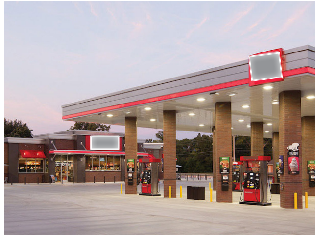
Example of C-Store Canopy
