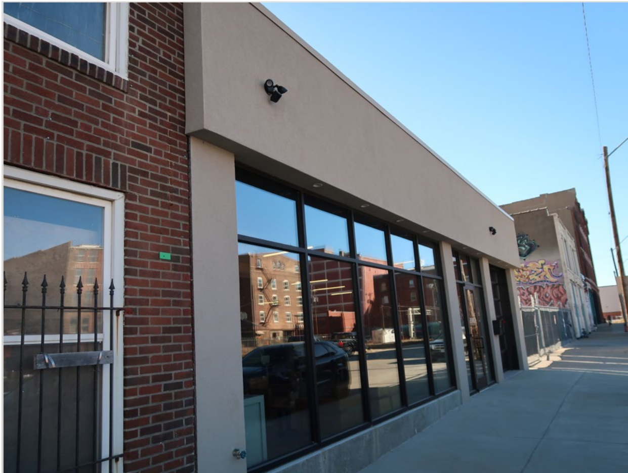
Looking Southwest At The Front (North) Elevation Of 1309 Union Avenue
