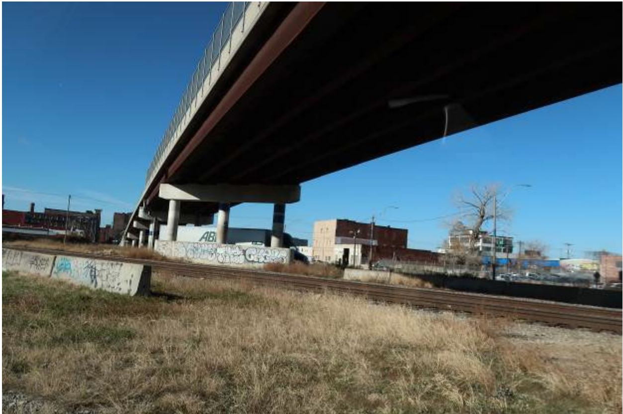
Looking Northwest Across 912 Santa Fe Street
