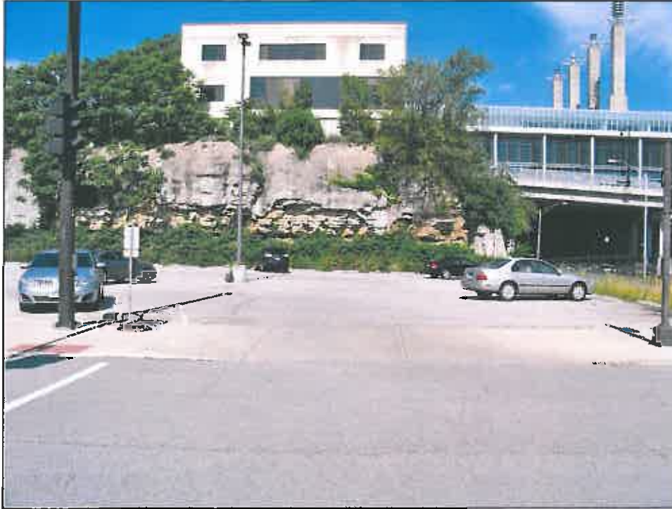
1514 Baltimore Avenue – inadequate signage and markings; parking stalls to right of entrance too close to entrance
