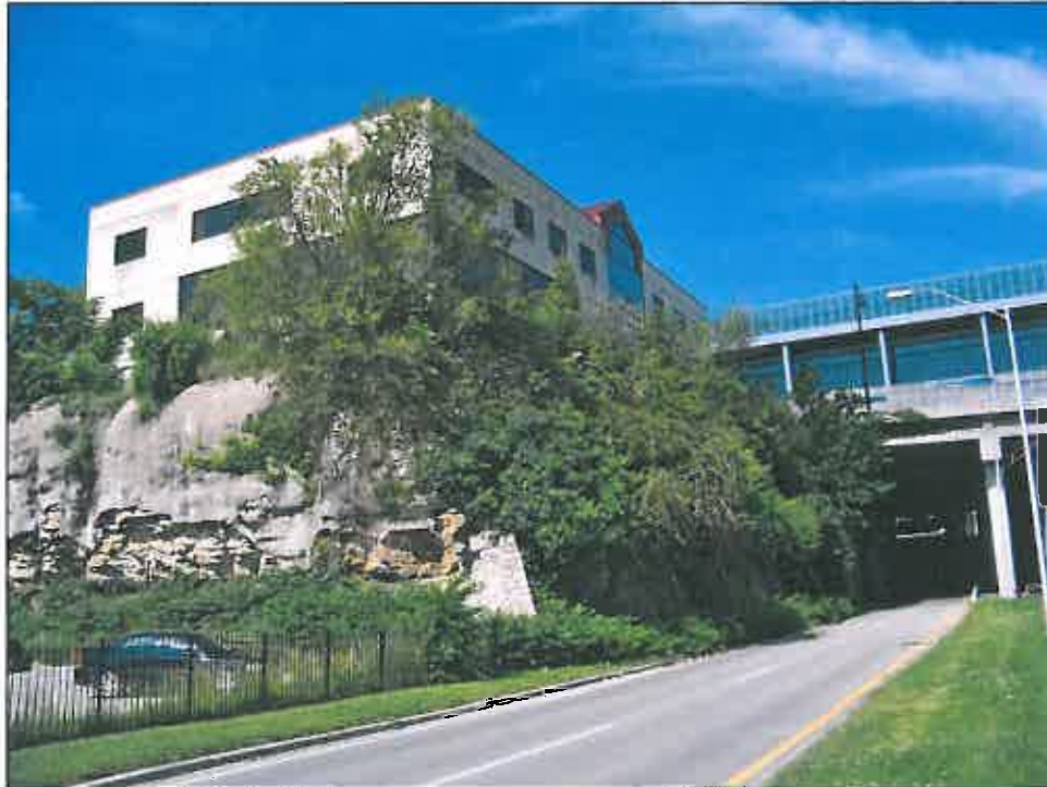
1514 Baltimore Avenue and 1501 Wyandotte Street – looking west – overgrown vegetation
