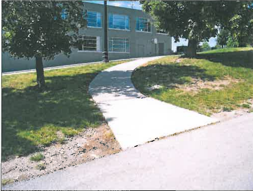
1514 Baltimore Avenue – looking southwest – lack of landscaping
