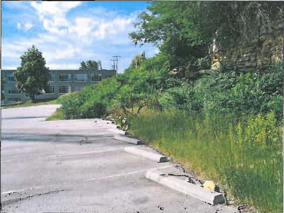
1514 Baltimore Avenue – looking south – overgrown vegetation; trash/debris; falling rock
