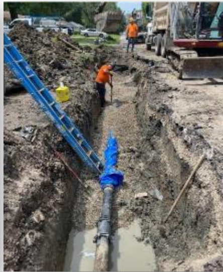
Supporting a New Water Main Section
