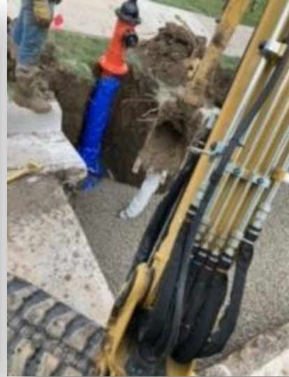
Installing a New Fire Hydrant
