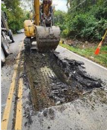
Excavator Digging up a Water Main Break
