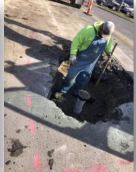
Adjusting a Valve Standpipe
