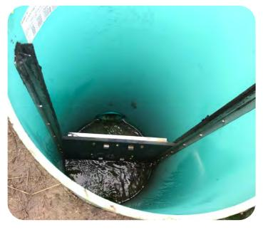
Inspect structural condition of pipe components. Check for damaged or broken pipes, pipe connections, or other underground features. Report any observed damage to the Owner. Verify that access points to underground features are present and secured in their proper place. If guards, covers or lids are missing, notify Owner.
