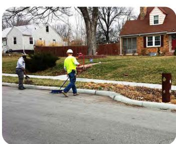
Remove sediment accumulation along perimeter of GSI if sediment is blocking water from entering. Check for erosion along perimeter and immediately upstream of component.
