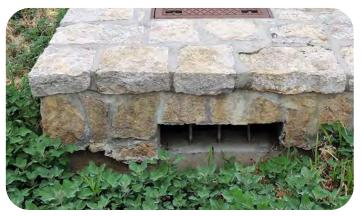
Inspect, clean, and exercise outlet control mechanism to assure it is properly functioning and that stormwater can enter pipe/manhole freely. If necessary, remove outlet control mechanism and remove any blockage in the pipe. Follow manufacturer's maintenance instructions, as applicable.
