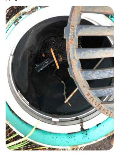
Remove and dispose of any blockages obstructing flow. If necessary, remove outlet control mechanism to remove blockages. Follow manufacturer's maintenance instructions, as applicable.
