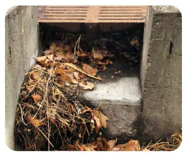
Remove any blockages within the structure. Clean or replace filter bag/basket, as necessary. Follow manufacturer's maintenance instructions, as applicable.
