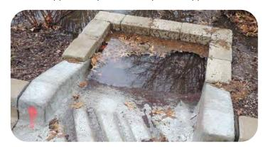
Inspect structural conditions of inlet. Check for loose or damaged inlets, grates or screens. Check for damaged or broken curbing or concrete structures. Report any observed damage to the Owner.
