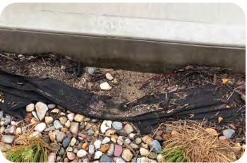
Fill small gullies with mulch or surface material. If erosion occurs in the same place more than one time, contact Owner. Fill larger gullies with decorative rock, appropriately sized for the permissible shear stress of stormwater entering the GSI, as directed by the Owner (see Green Stormwater Infrastructure Manual GSI-2.1). Check for mulch or soil slumping. Rake back into place.
