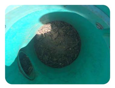
Inspect conditions of outlets. Check for loose or damaged outlets, outlet pipes, grates or screens. Check for damaged or broken curbing or concrete structures. Report any observed damage to the Owner.
