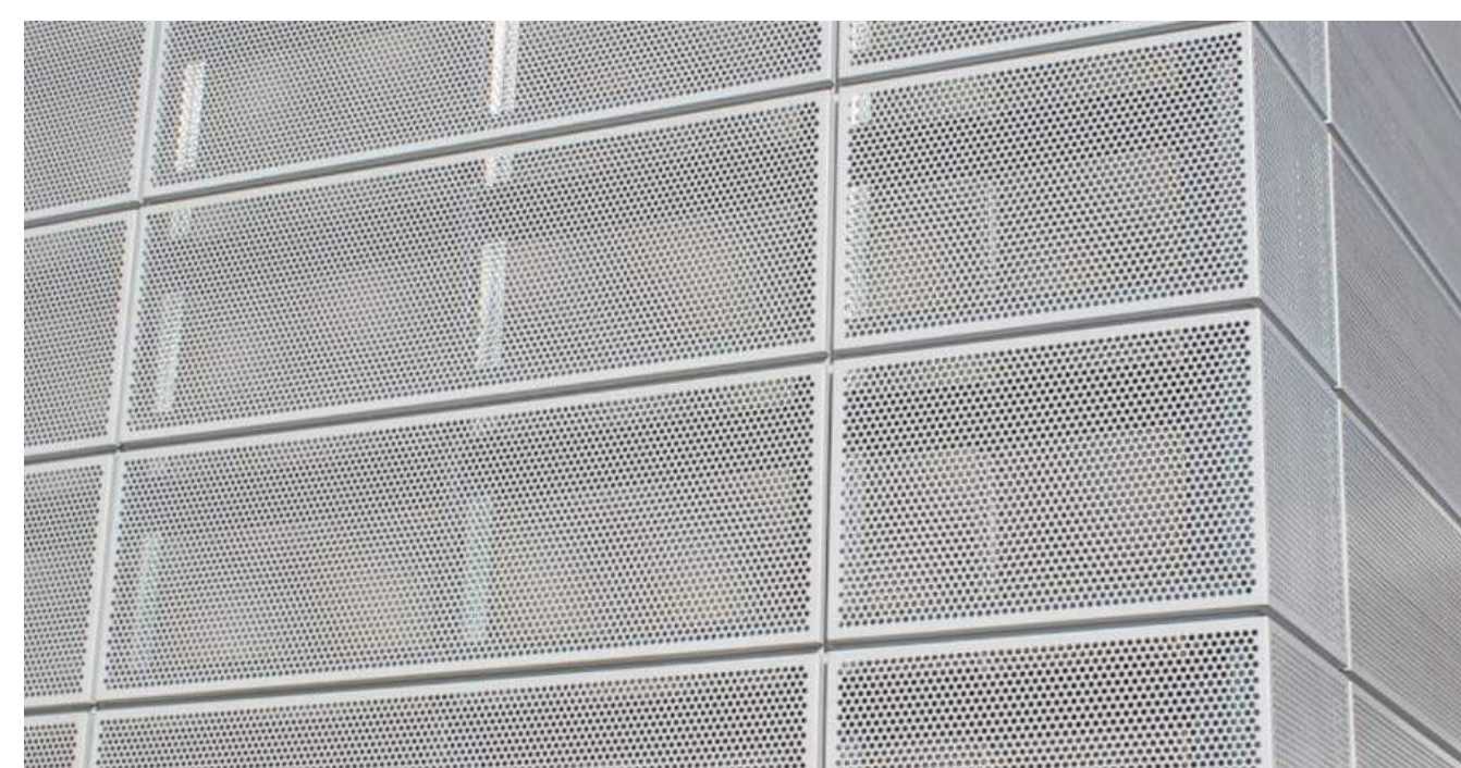
PERFORATED METAL SCREEN WALL / SUN SCREEN
