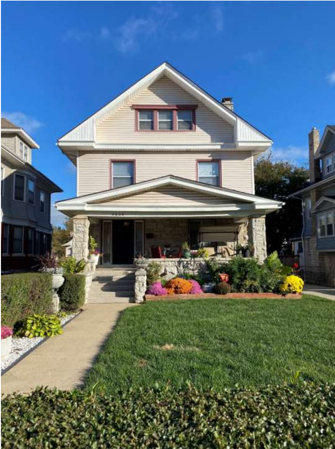
Front (South) Façade
