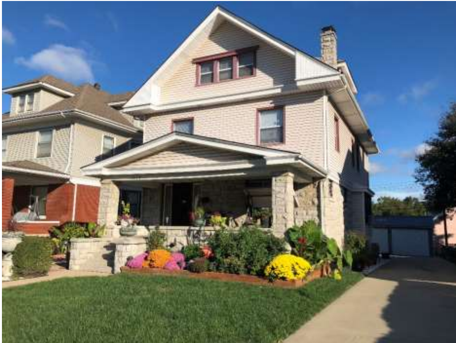
Front and East Facades
