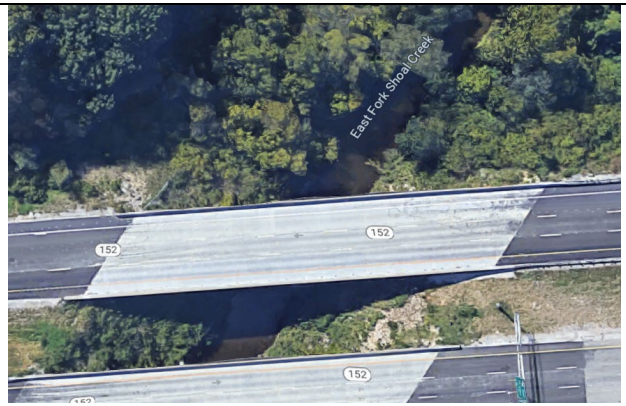
Aerial view Mo 152 and East Fork Shoal Creek
