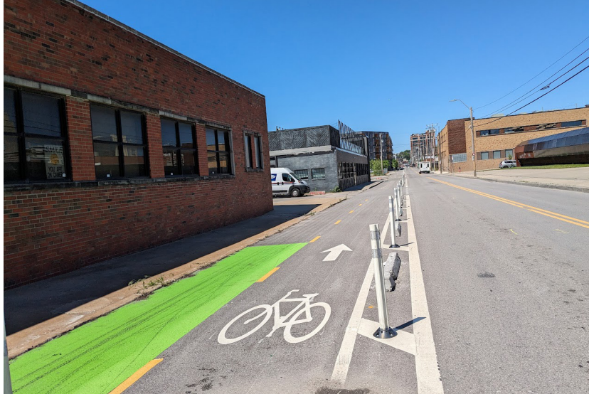
Figure 3 – Two-way cycle track using quick-build materials
