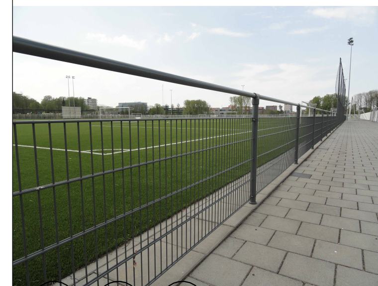
Proposed Fence Design Steel welded wire fence; painted black; transparency to be at least 80%
