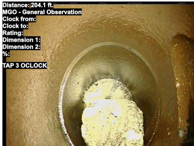
SHEET 25 S087-154 IS NOT A MANHOLE LISTED AS O/C POINT REPAIR BASE BID
