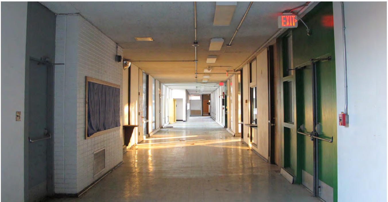
Photo of St. Francis Xavier School hallway - the light at the end of the tunnel.
